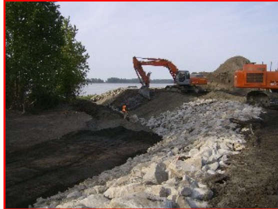
Native Sediments Placement Over Rip Rap
