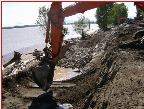
Bank Excavation and Shaping of Dike Toe
