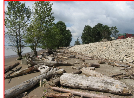
Arrangement of Logs at Dike Toe
